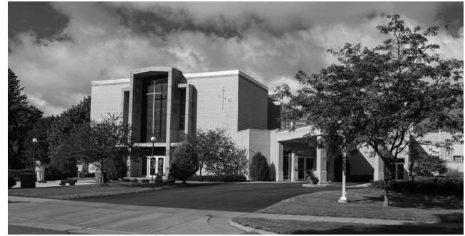
ST. JAMES THE GREATER PARISH 2502 11th Street | Eau Claire (715) 835-5887
